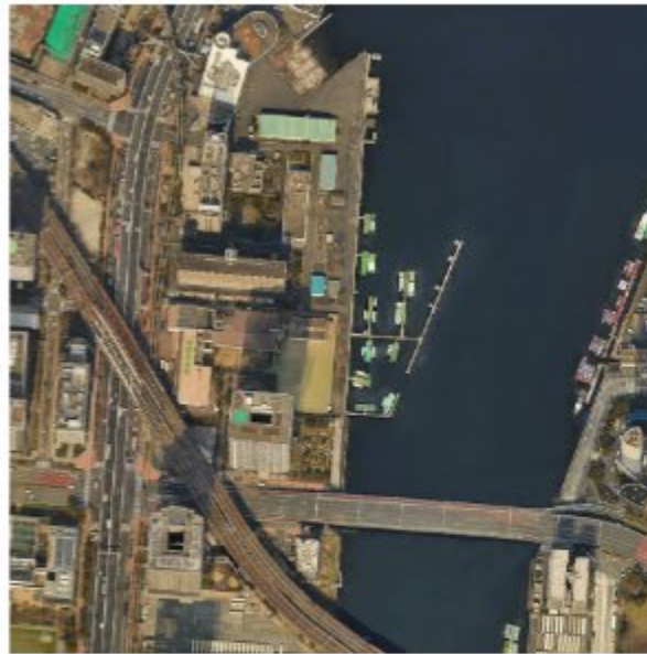
(b) Cross-river bridge.
